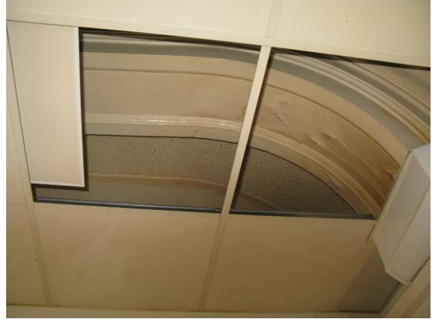
Moulded plasterwork to ceiling ribs above kitchen
