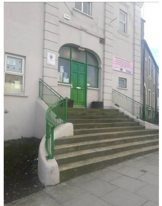
Sweeping entrance steps
