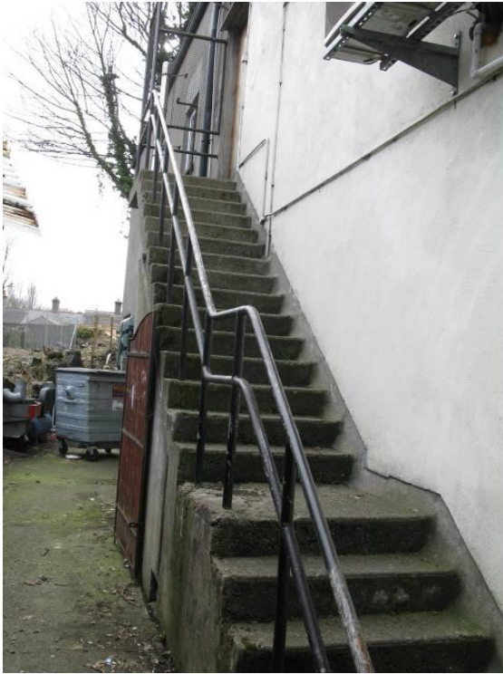
South side fire escape
