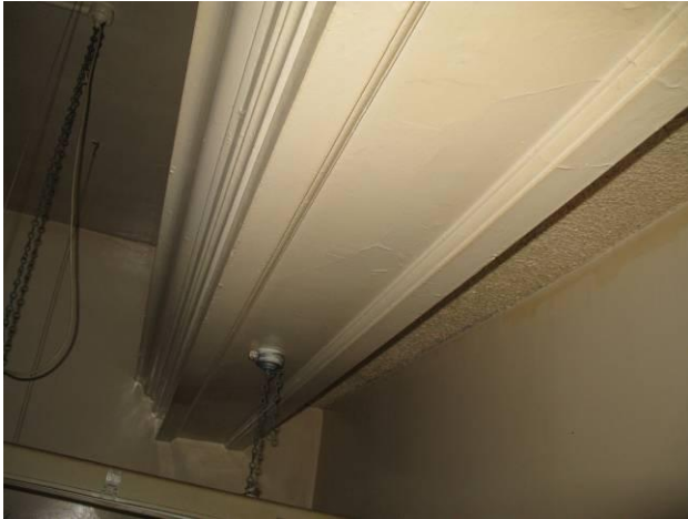
Cornice detail to auditorium ceiling adjacent to north wall.
