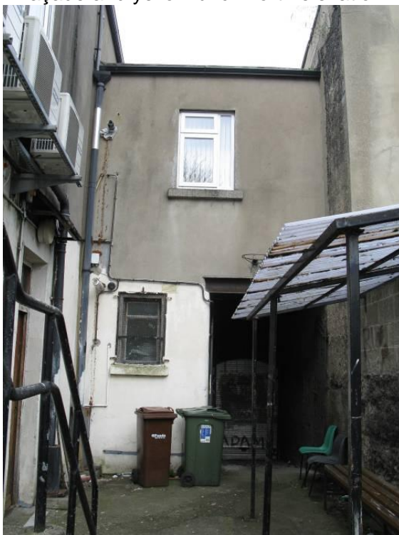
Rear elevation of two-storey extension
