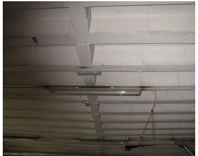
Ground floor inserted ceiling
