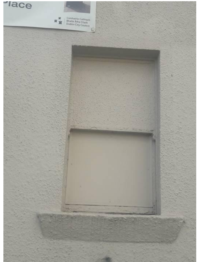
Original single pane timber sash window with distinctive chamfered cill
